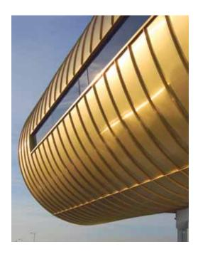
Nordic Royal™ is an alloy of copper with aluminium and zinc, giving it a rich golden through-colour and making it very stable. It has a thin protective oxide layer containing all three alloy elements when produced. As a result, the surface retains its golden colour and simply loses some of its sheen as the oxide layer thickens with exposure to the atmosphere to give a matt finish. It behaves differently to other Aurubis copper products over time and does not develop a blue or green patina.
