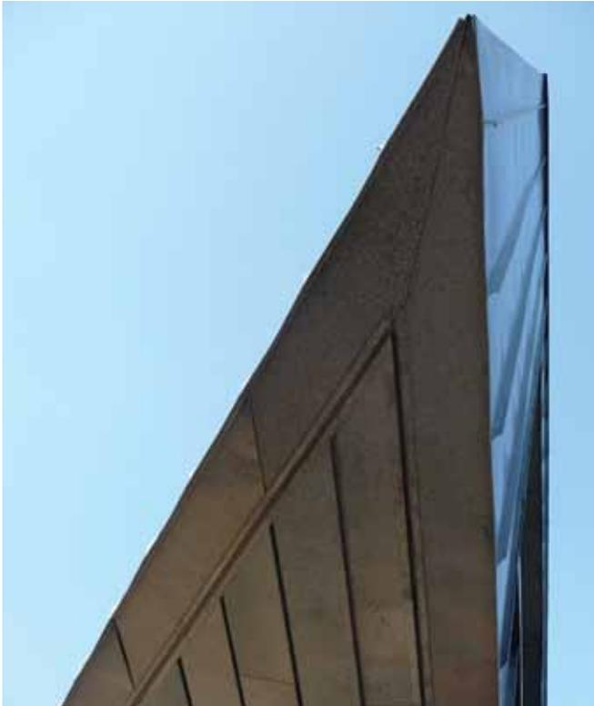
The most common compound found in natural patinas all over the world is the copper sulphate mineral brochantite. Aurubis' factory-applied patinas have been developed with properties and colours based on the same brochantite mineralogy.
